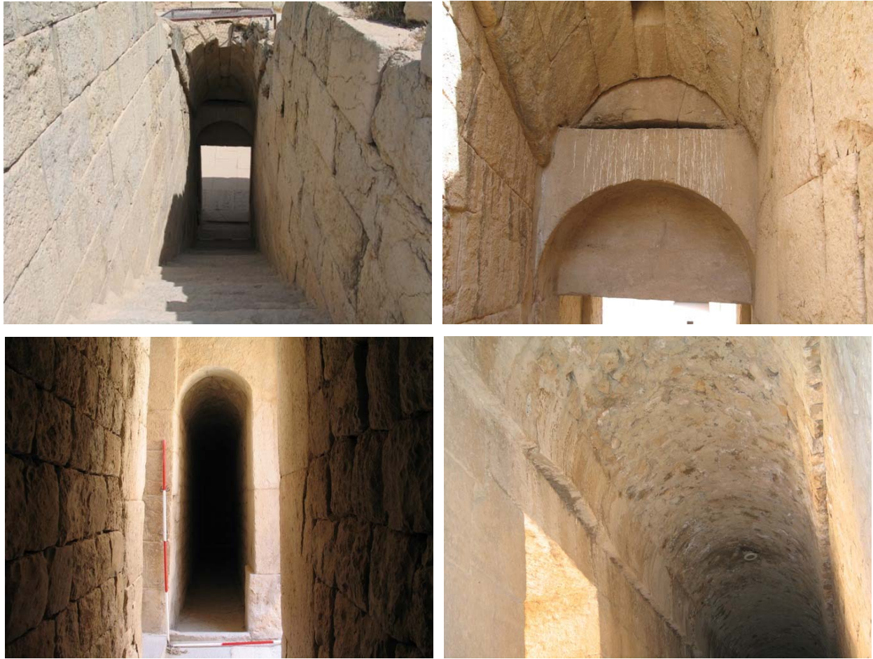
Fig.2-8. Cradle vault in Anahita Temple, Photo by the author.
