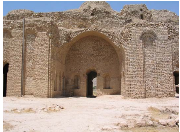
Fig. 2-4. Various vaults and arches in Ardashir I, Palace (3 rd century AD.), Barrel vault, Horseshoe arch, Firuzabad, Photo by the author.
