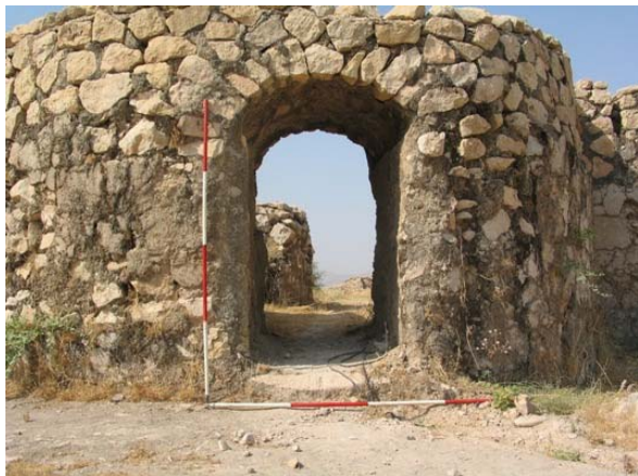
Fig. 2-7. Semi-circular vault and arch on the wall of the city of Bishapur , Photo by the author.
