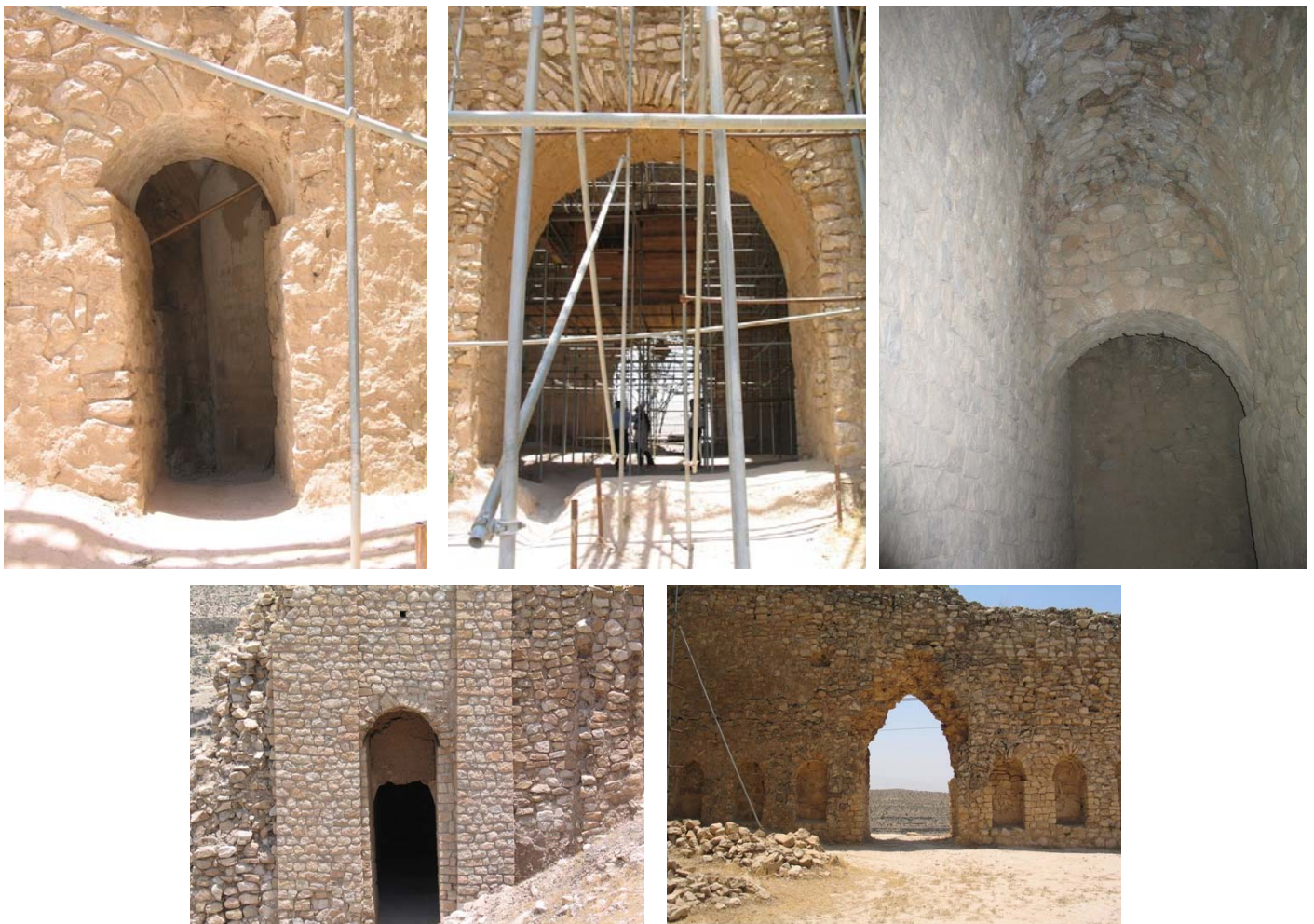
Fig. 2-3. Barrel vault, cradle vault, horseshoe vault and arch Qal'a-yi Dukhtar, Firuzabad (3 rd century AD), (Photo by the author).
