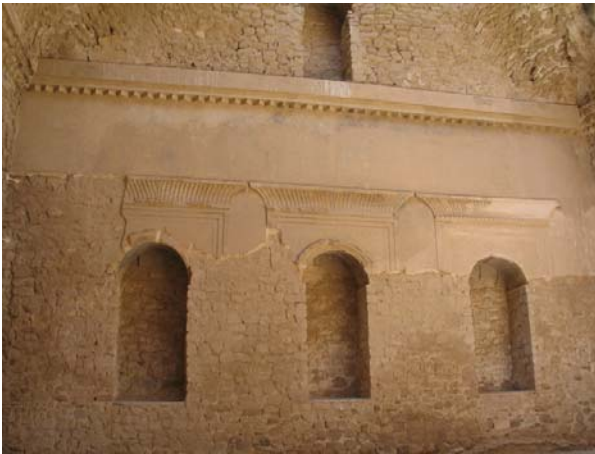
Fig. 2-4. Various vaults and arches in Ardashir I, Palace (3 rd century AD.), Barrel vault, Horseshoe arch, Firuzabad, Photo by the author.
