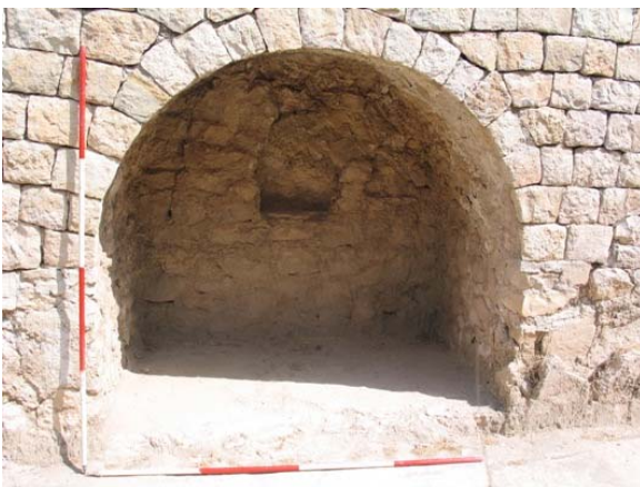
Fig. 2-7. Semi-circular vault and arch on the wall of the city of Bishapur , Photo by the author.
