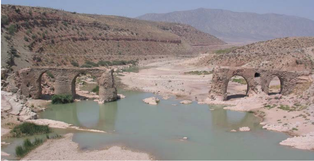
Fig. 2-2. Application of semi-circle arch in Firuzabad Bridge, (Photo by the author).
